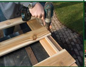
Measure distance between top and bottom board. Place two other rails and space equally. Cut two scraps to ensure the accurate placement of the horizontal rails.
