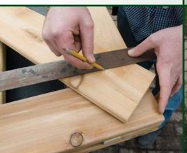
Using a straight edge mark pencil line on diagonals even with inside edge of stiles. Mark top and bottom. Remove top rail and diagonal. Cut along pencil marks.
