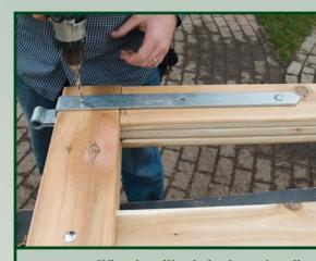
When installing bolts do not install bolts at top corner where hardware will attach. Center hardware on rails, drill holes and attach with fasteners provided.
