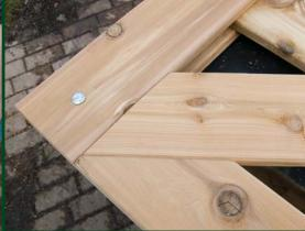
Lay top rail and diagonal in place ensuring a good ft. Install a 1.5" wood screw into each (screwing up from the bottom) to hold top rail and diagonal in place.
