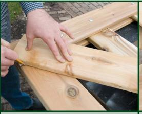
Lay diagonal braces on surface (allow 1/2" from top of top rail) Mark top rail with pencil line.
