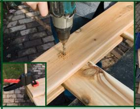
Turn the gate over. Attach second stile at each end. Use 3.5" x 3/8" galvanized carriage bolts. Tip: use quick clamps to hold stiles in place while drilling.
