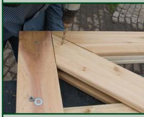
Turn the gate over and repeat steps 5 thru 8 on the other side. Drill a hole at each intersection point and install 3.5" x 3/8" galvanized carriage bolt at each location.
