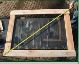
Measure the two diagonals and adjust gate so that they are equal (this will ensure the gate is square). Install another 1.5" fastener at each inside corner.
