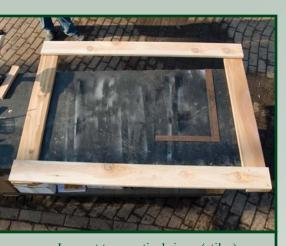
Lay out two vertical risers (stiles), to rail and bottom rail in rectangular shape. Fasten each of the outside corners with a single 1.5" wood screw.
